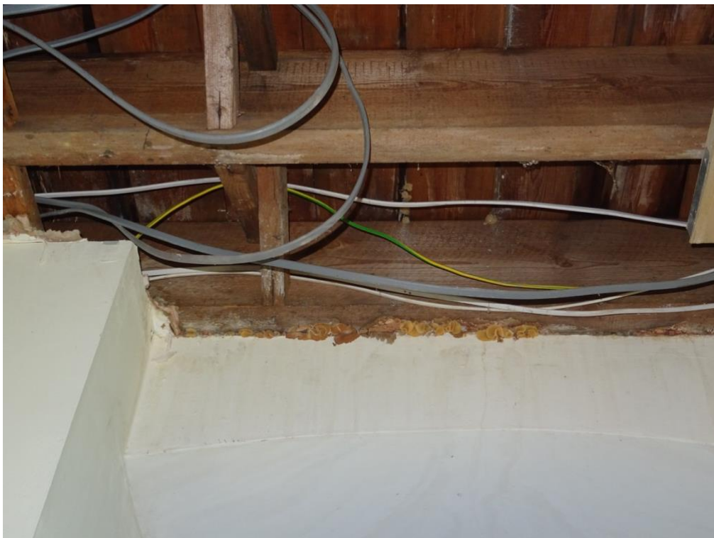
Figure 20 Fungal growth to supporting timbers
