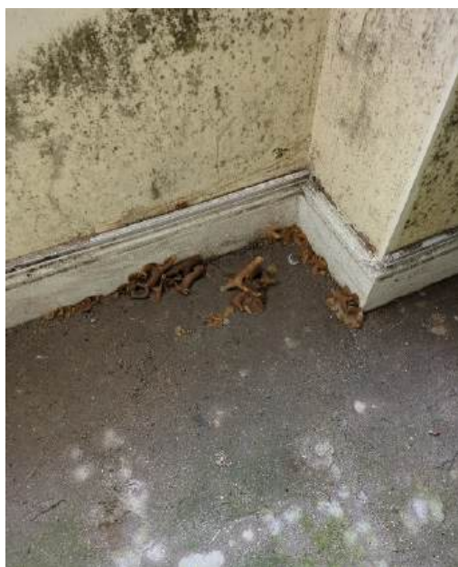
Photograph 35 - Fungal growth on lounge concrete floor (GF Horseshoe cottage)
