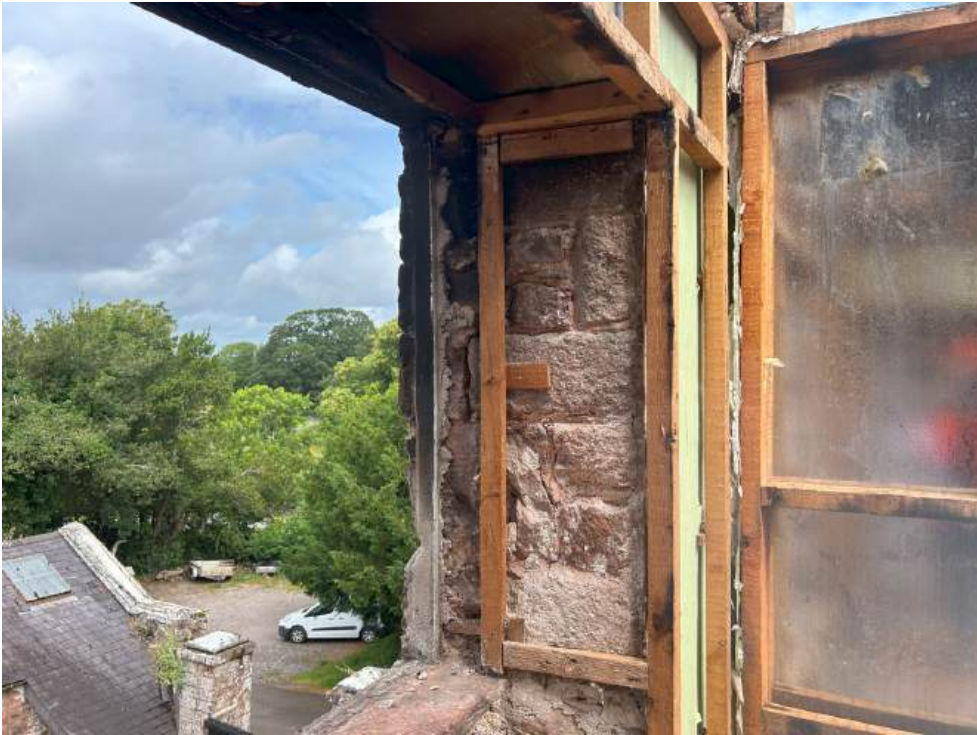
Photograph 5 - 550mm thick external stone walls.
