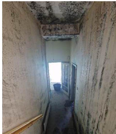
Photograph 12 - Hallway wall finish covered in mould (LGF Yew tree cottage)
