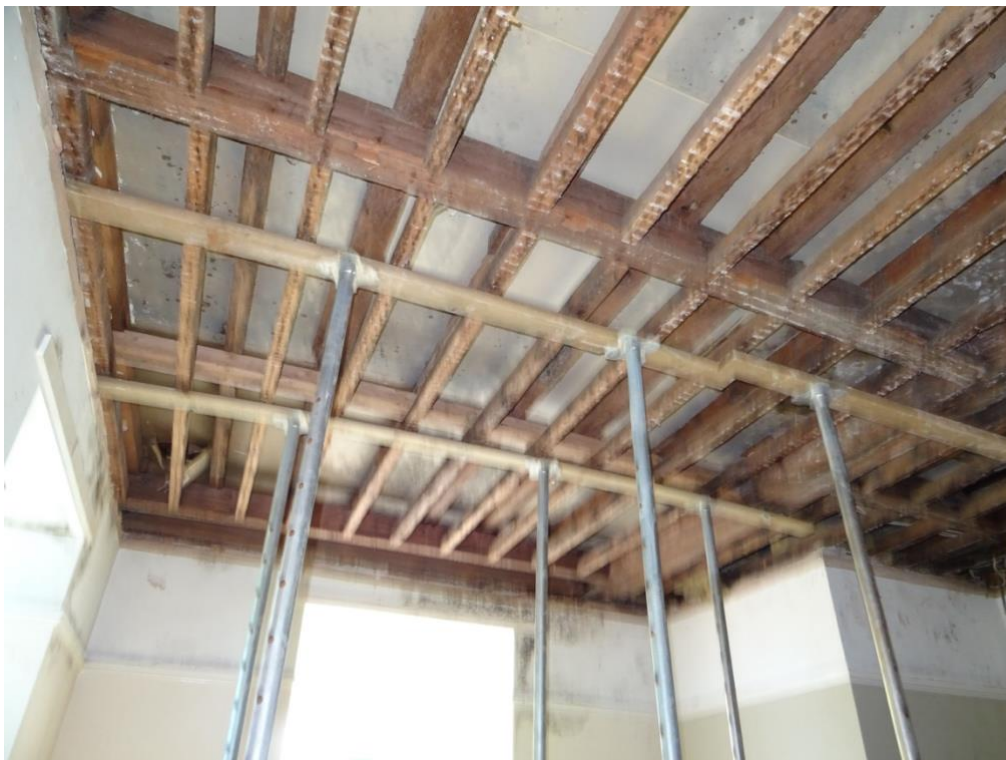
Figure 22 Supporting props to first floor structure.
