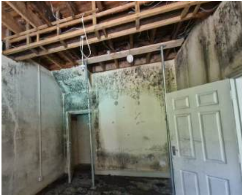
Photograph 5 - Significant mould growth on walls (LGF Yew tree cottage)
