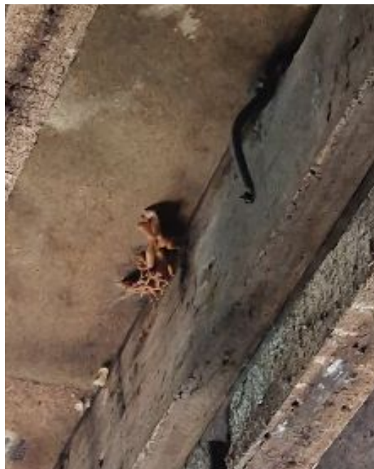
Fig. 15. Photo 7 - Fungal growth observed to timber suspended floor
