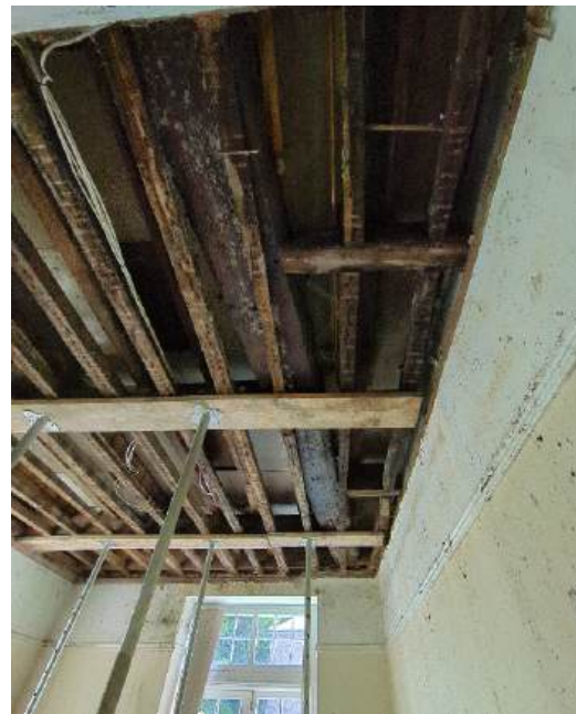
Photograph 40 - Bedroom 1 ceiling finish removed (GF Horseshoe cottage)
