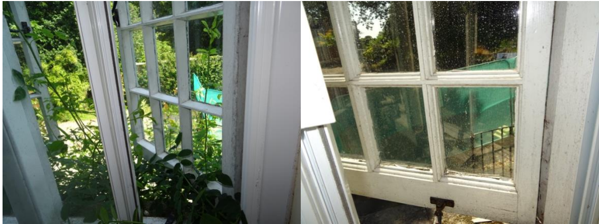
Figure 23 An example of the different glazing bar styles within the property.
