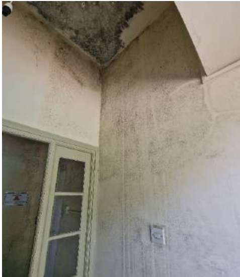
Photograph 9 - mould growth on wall (LGF Yew tree cottage)
