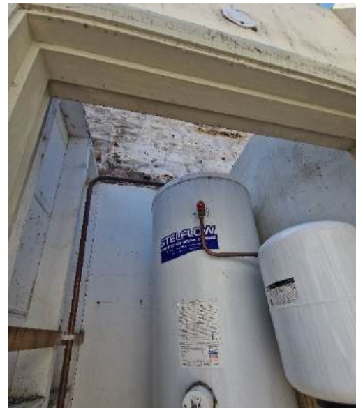
Photograph 16 - No ceiling finish in immersion cupboard (GF Yew tree cottage)
