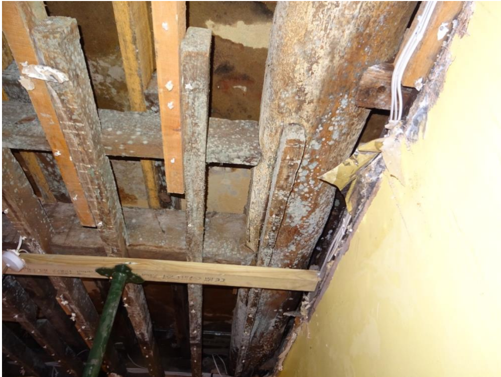
Figure 21 Mould and damp to supporting timbers
