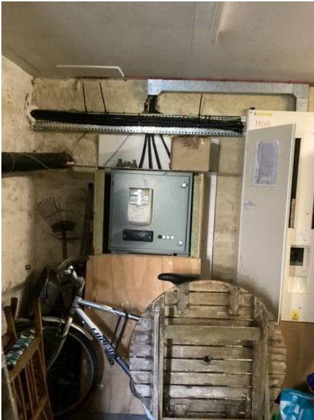
Photograph 83 - Electrical Mains Incomer & Panel Board To Commercial Units
