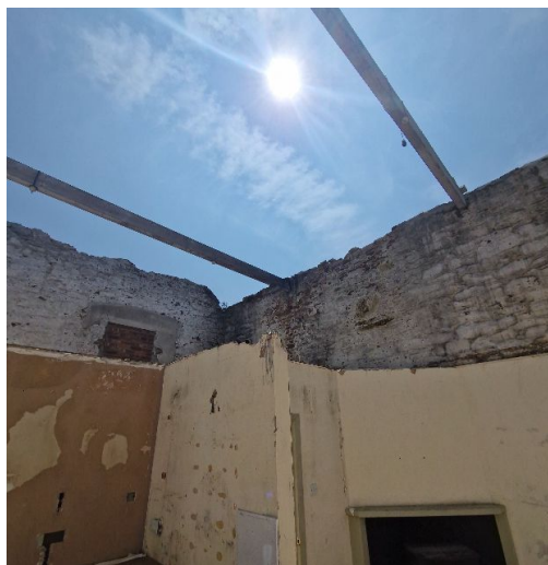
Fig. 9. Photo 1 - Roof removed due to extensive fire damage
