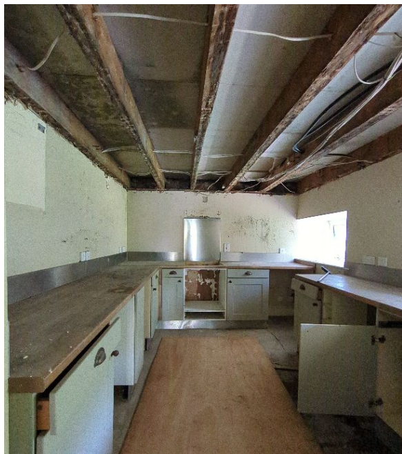
Fig. 14. Photo 6 - Horseshoe Cottage, Kitchen ceiling finish removed
