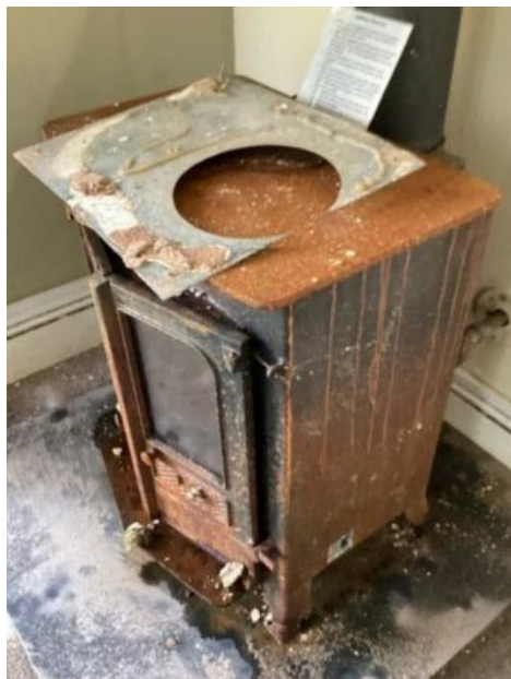
Fig. 23. Photo 15 - Horseshoe Cottage, Wood burner heavily corroded
