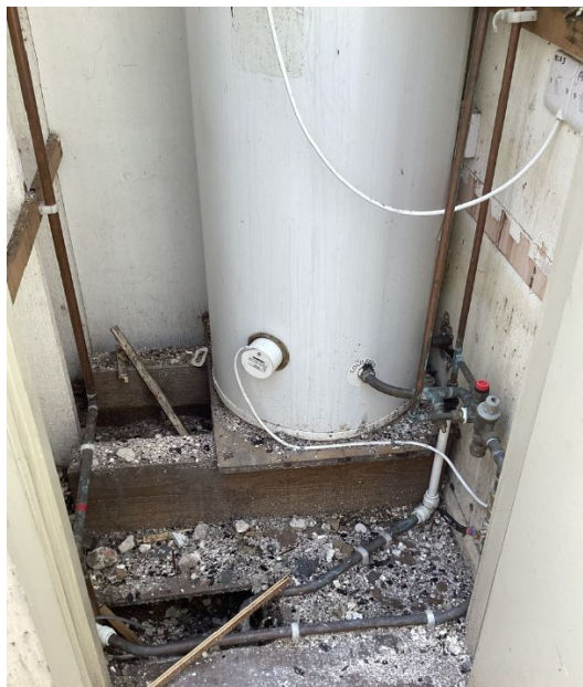
Fig. 21. Photo 13 - Yew Tree Cottage, Immersion heater likely water damaged
