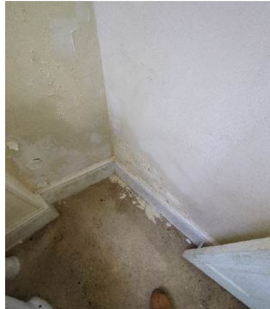
Photograph 30 - bathroom walls damp (LGF Horseshoe cottage)
