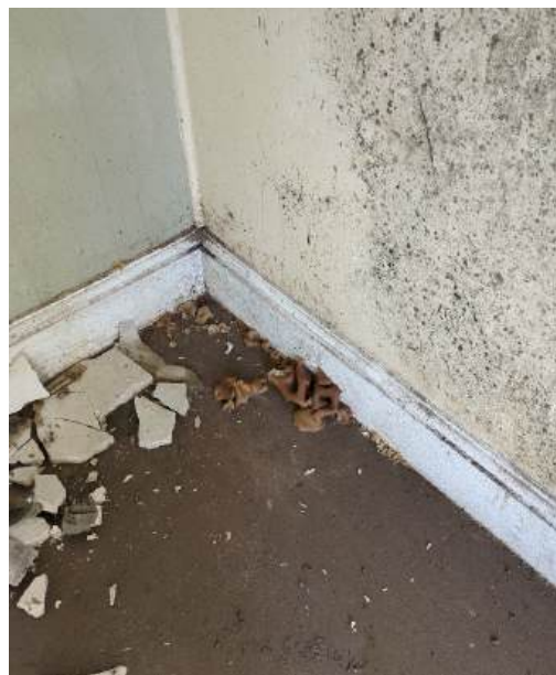
Photograph 42 - Fungal growth around skirting in bedroom 1 (GF Horseshoe cottage)
