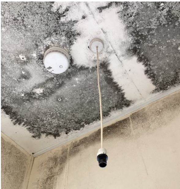
Fig. 17. Photo 9 - Water damaged Upvc ceiling rose and cable
