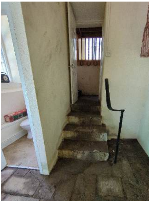
Photograph 31 - Concrete staircase heavily stained (LGF Horseshoe cottage)
