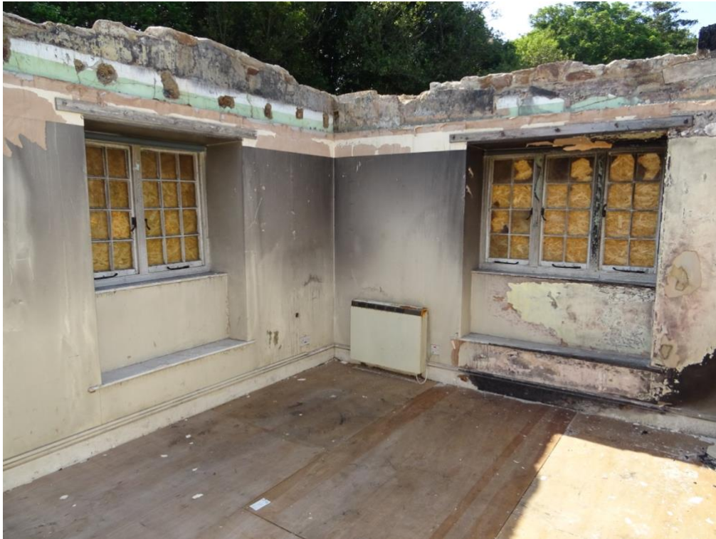
Figure 15 Damaged and undulating wall head. Also damaged and boarded windows.
