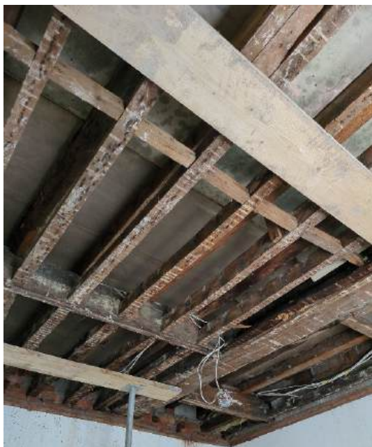
Photograph 43 - Bedroom 2 ceiling finished removed (GF Horseshoe cottage)
