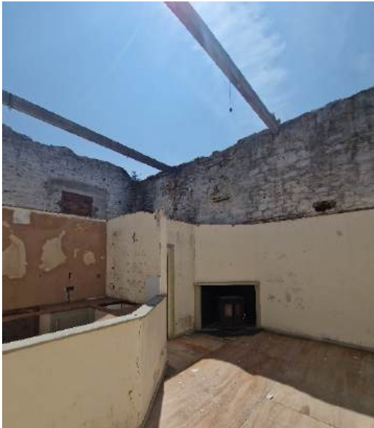
Photograph 13 - No ceiling in kitchen (GF Yew tree cottage)
