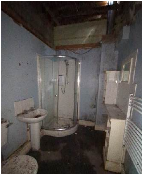
Photograph 37 - Sanitary units heavily stained (GF Horseshoe cottage)
