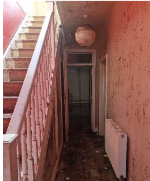
Photograph 22 - Staining to hallway walls (GF Flat 6)
