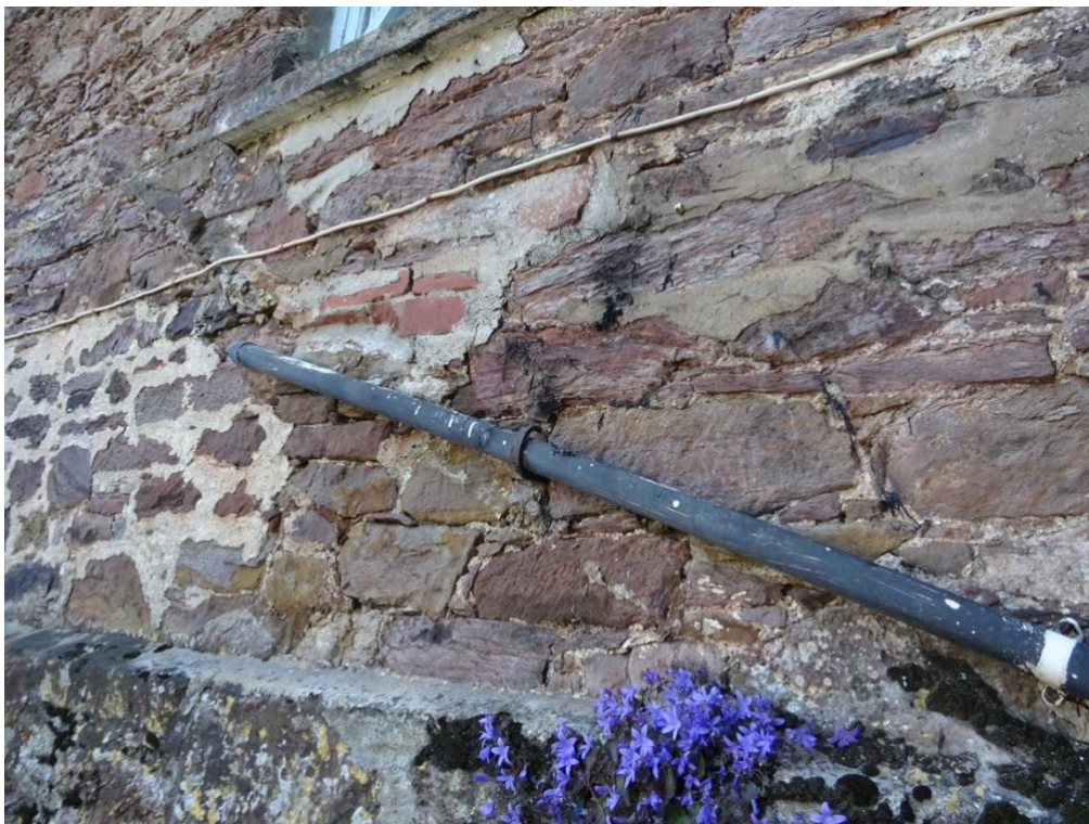
Figure 28 Poor cement based mortar to walling.
