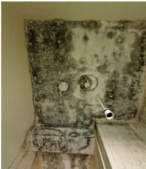
Photograph 11 - Hallway ceiling finish covered in mould (LGF Yew tree cottage)
