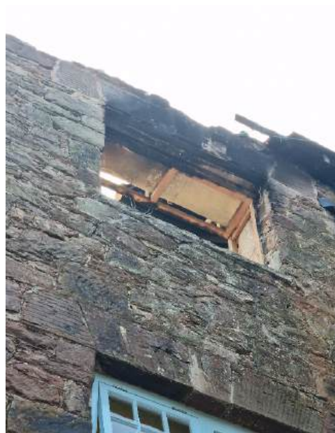
Photograph 68 - blown out window (West elevation)
