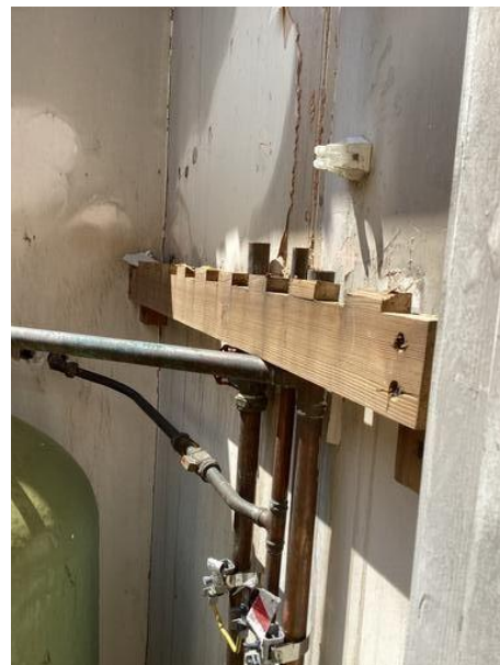
Photograph 58 - Flat 6 (Immersion) Pipes To Above Cut Off
