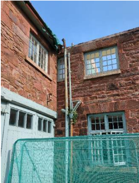
Photograph 65 - Disconnected downpipes (South elevation)
