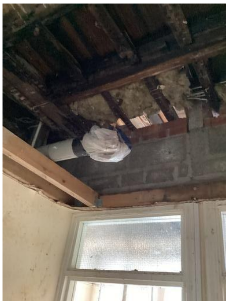
Photograph 31 - Horseshoe Cottage (Hall) Ventilation Duct (Assumed)
