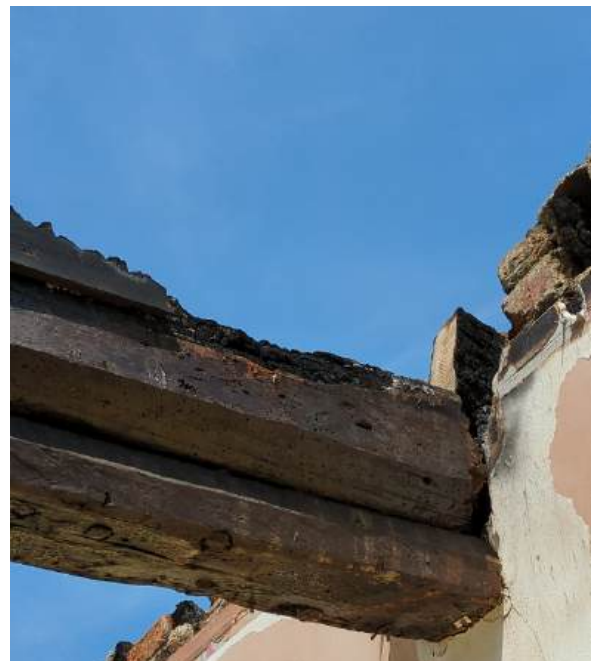
Photograph 56 - significant charring to timber truss in bedroom 3 (1F flat 6)
