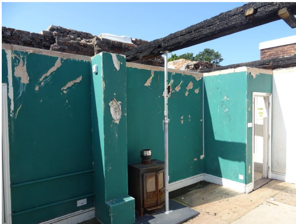
Figure 17 Retained chord tie beam.
