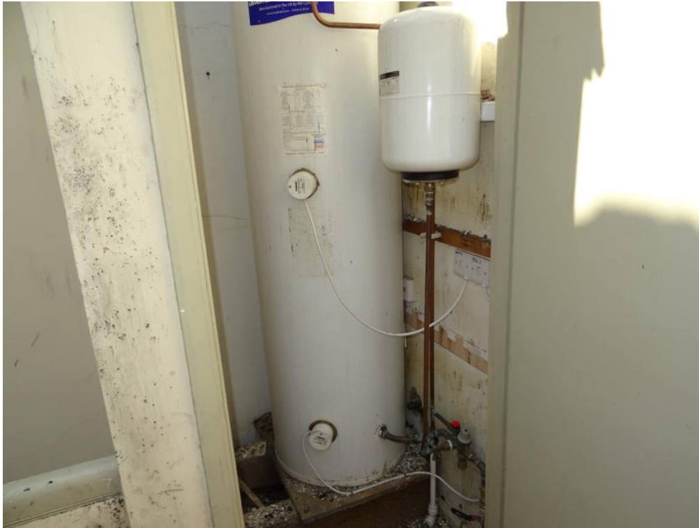
Figure 27 Example of hot water system to the apartments.
