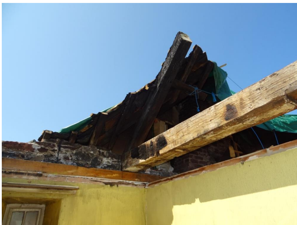
Figure 18 Retained chord tie beam.
