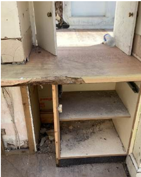
Photograph 47 - kitchen units damaged ((1F Horseshoe cottage)
