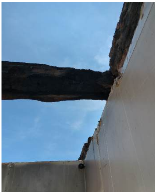
Photograph 49 - Timber roof truss heavily charred (1F Horseshoe cottage)
