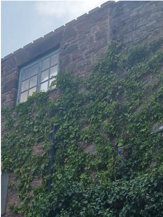
Photograph 69 - Disconnected downpipes (West elevation)
