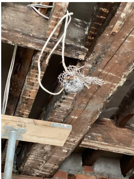
Photograph 39 - Horseshoe Cottage (Bed 2) General Wiring & Smoke Detector
