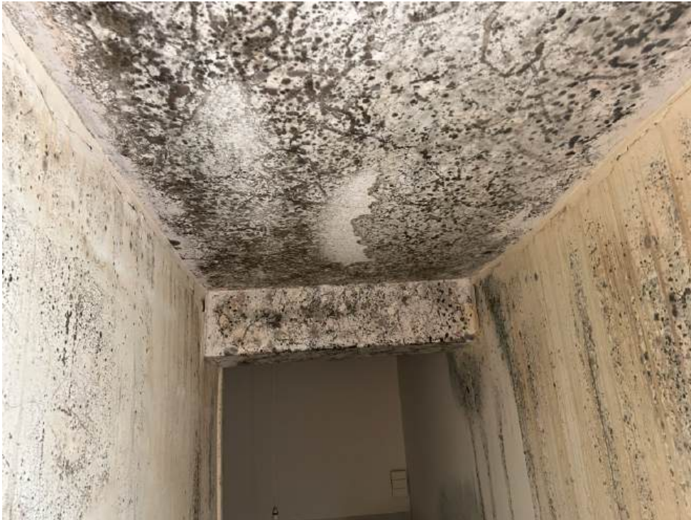
Photograph 8 - Damp to walls and ceiling.
