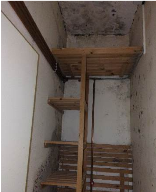
Photograph 45 - Airing cupboard ceiling finish moldy (GF Horseshoe cottage)
