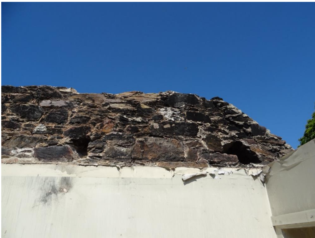
Figure 16 Fire damaged wallhead.
