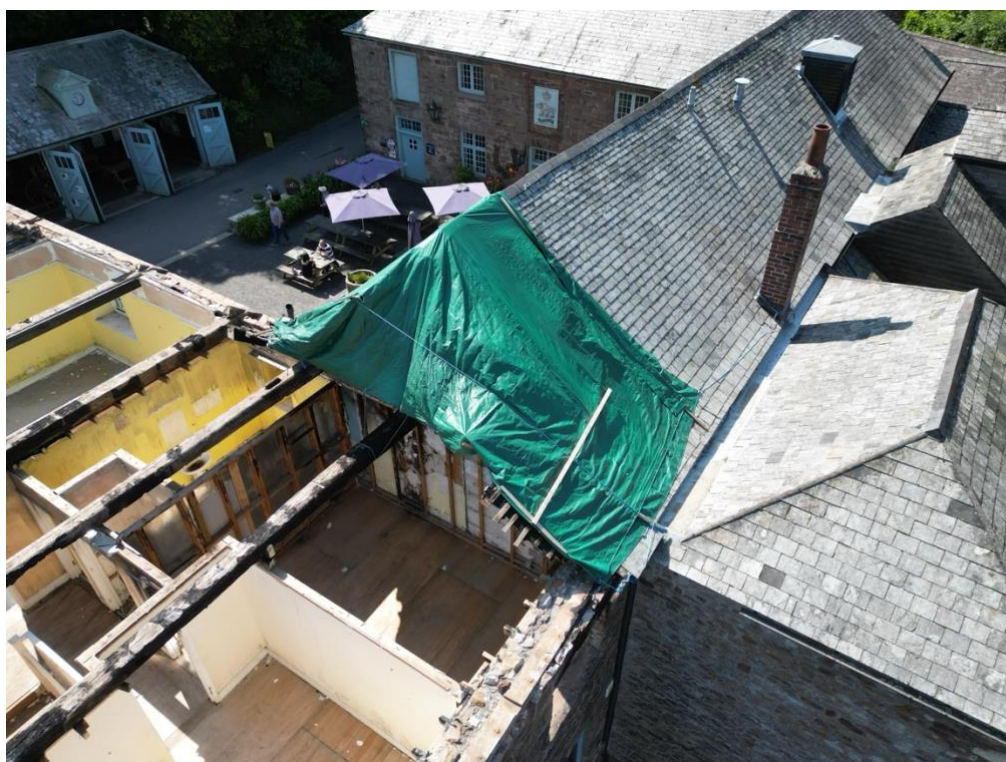
Figure 10 Abutment to central wing where further spread of the fire was prevented.
