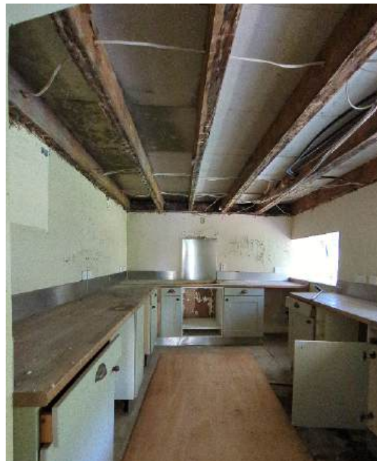
Photograph 32 - kitchen ceiling finish removed (GF Horseshoe cottage)
