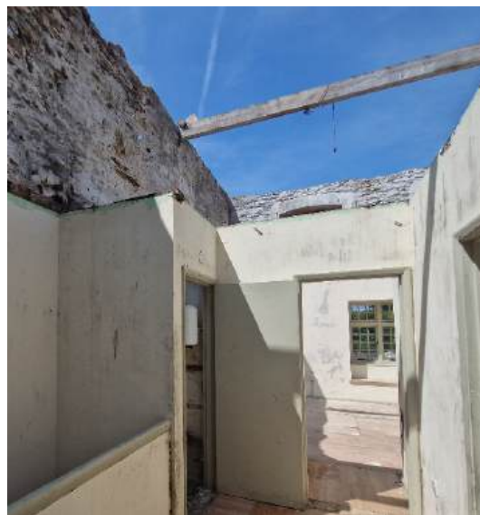
Photograph 18 - No ceiling in hallway (GF Yew tree cottage)
