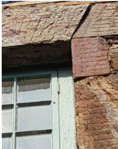
Fig. 12. Photo 4 - Stone lintel to North East corner displaced
