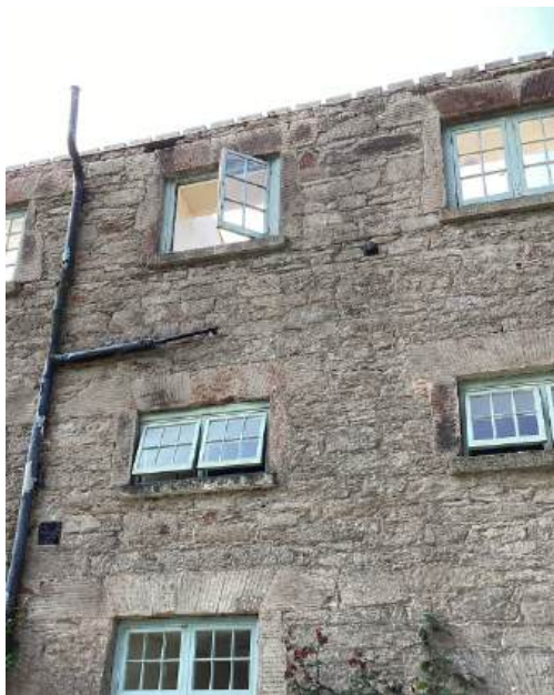
Photograph 59 - Staining to key stones (North elevation)
