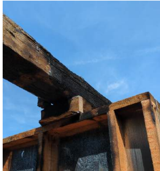
Photograph 54 - Significant charring to the timber truss in bedroom 2 (1F flat 6)
