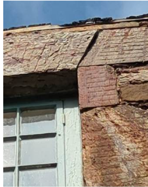
Photograph 62 - Key stone misalignment (East elevation)
