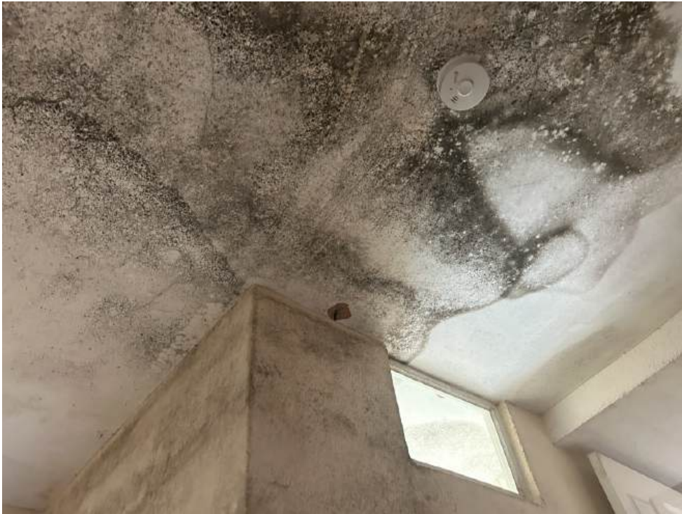
Photograph 9 - Damp to walls and ceiling
