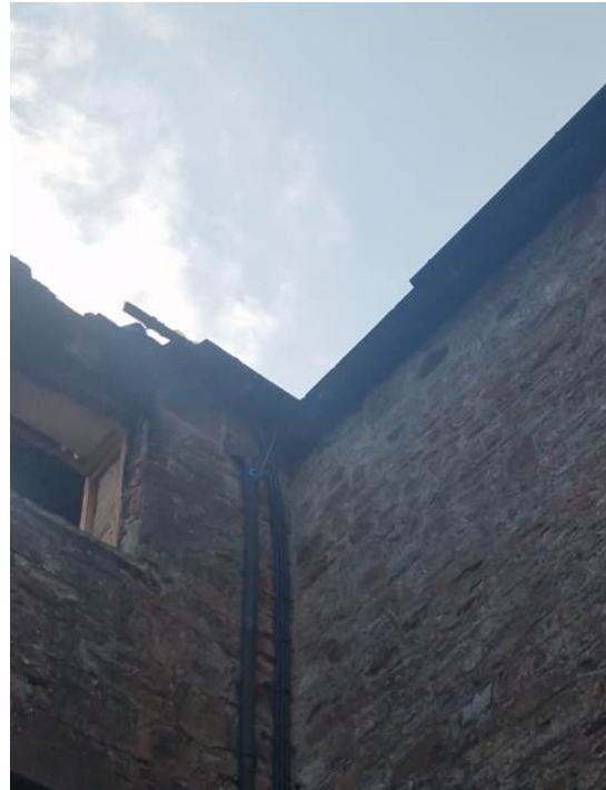
Photograph 70 - Disconnected guttering (West elevation)
