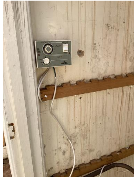
Photograph 60 - Flat 6 (Immersion) Control
