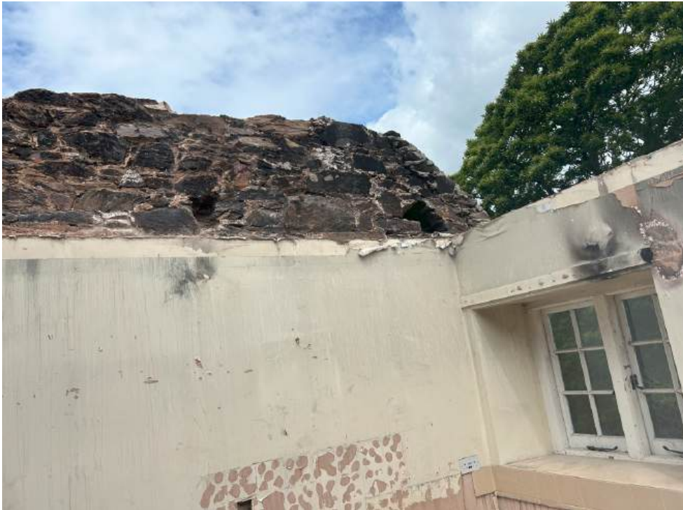
Photograph 10 - Missing stone blocks.
