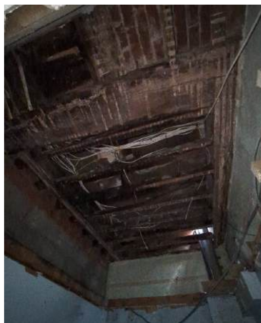
Photograph 36 - bathroom ceiling finish removed (GF Horseshoe cottage)
