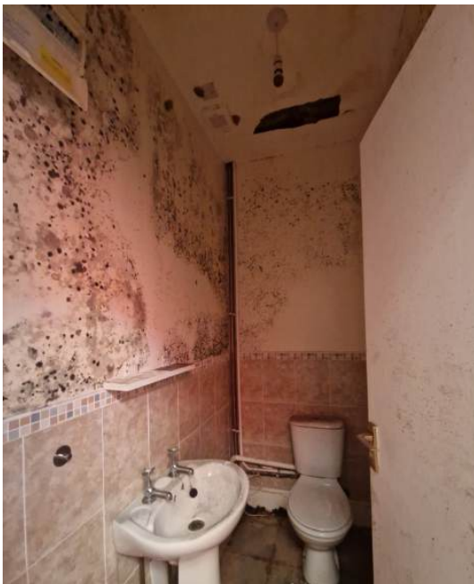
Photograph 27 - bathroom wall finishes mouldy (GF Flat 6)
