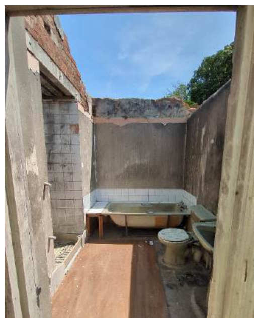
Photograph 52 - Sanitary units are smoke stained (1F Horseshoe cottage)
