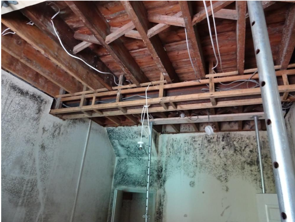
Figure 19 Ceiling areas removed from much of the lower floors.
