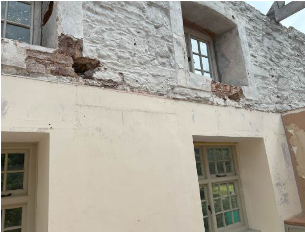
Photograph 7 - Missing stone blocks.
