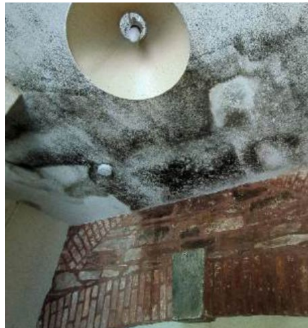
Fig. 16. Photo 8 - Horseshoe Cottage, black mould on lobby ceiling
