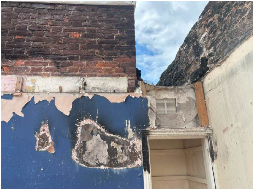
Photograph 11 - Charred timber embedded in stone wall..
