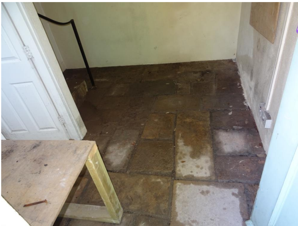
Figure 25 Retained stone flag floor to Horseshoe Cottage.
