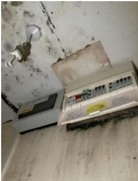
Fig. 20. Photo 12 - Distribution board water damaged
