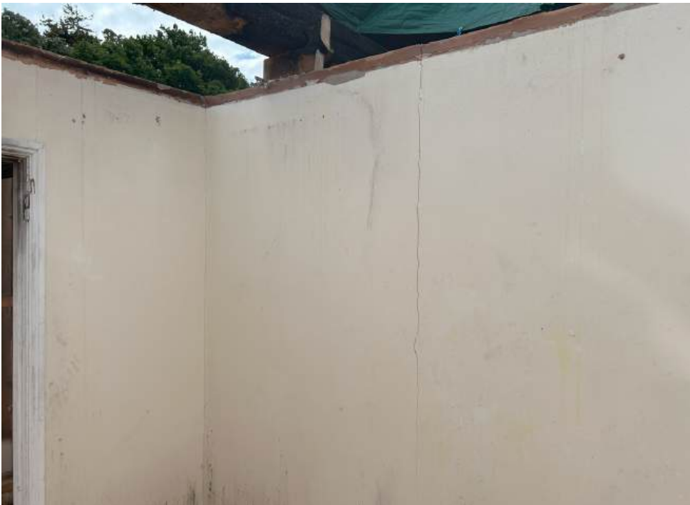
Photograph 6 - Crack to plaster finishes at first floor.
