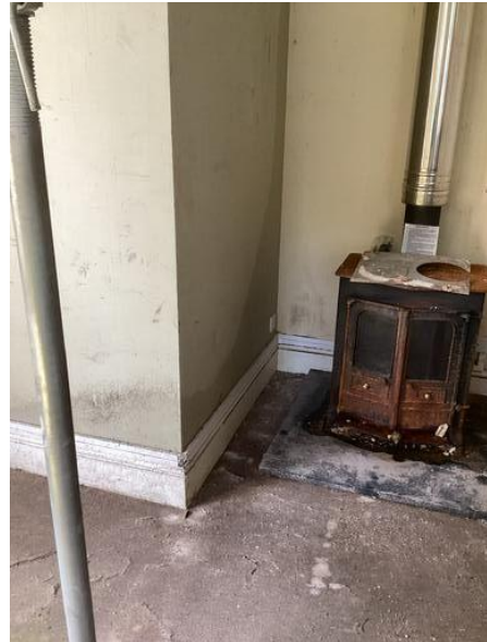
Photograph 20 - Horseshoe Cottage (Lounge) Wood Burner With Back Boiler
