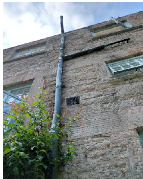
Photograph 60 - Decorative wear to SVP (North elevation)
