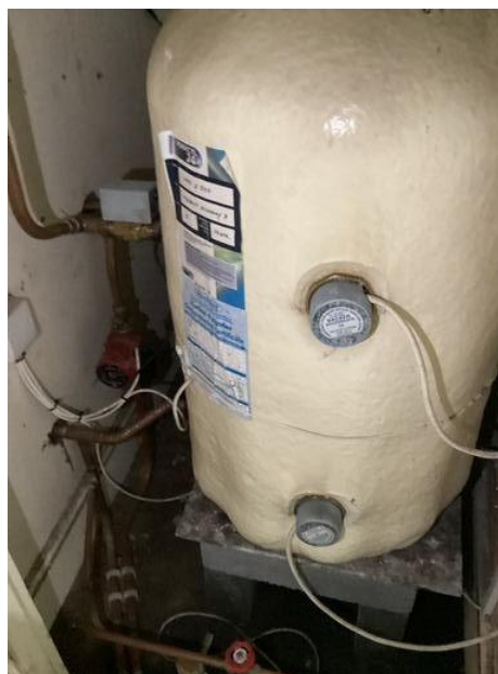
Photograph 26 - Horseshoe Cottage Immersion Cylinder
