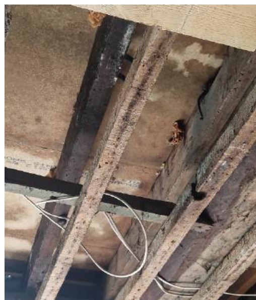
Photograph 18 - No ceiling in hallway (GF Yew tree cottage)
