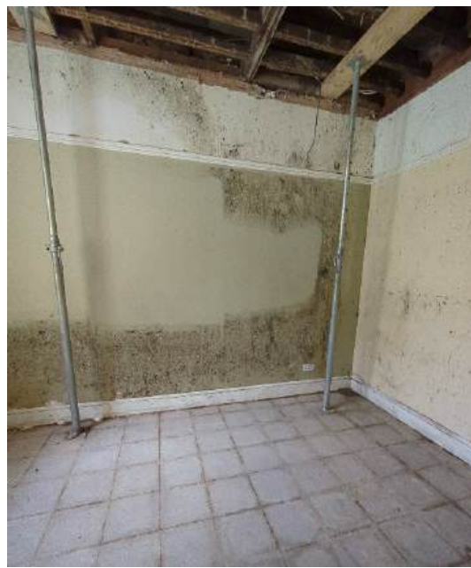
Photograph 44 - Bedroom 2 wall finish stained (GF Horseshoe cottage)
