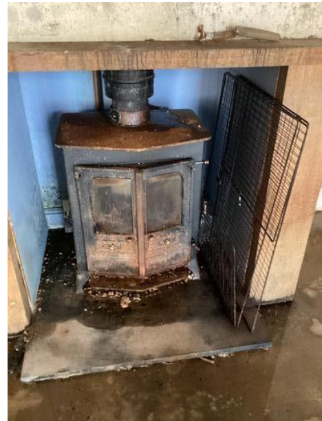
Photograph 54 - Flat 6 (Lounge) Wood Burner With Back Boiler
