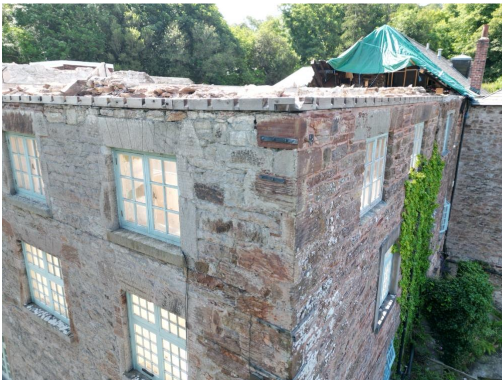
Figure 12 North west corner. The crenulated soffit design can be seen here which should be replicated moving forward.
