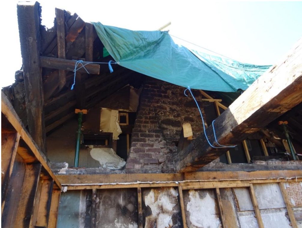
Figure 11 Abutment to central wing where further spread of the fire was prevented.
