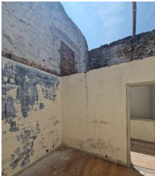
Photograph 15 - No ceiling finish in bedroom 1 (GF Yew tree cottage)
