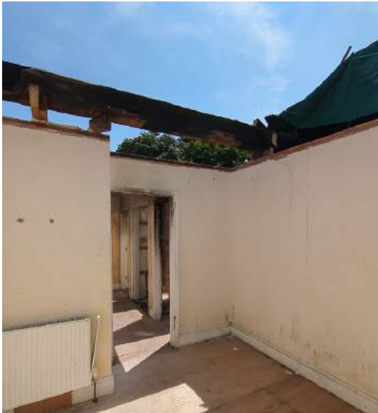
Photograph 53 - Significant charring to the timber truss in bedroom 1 (1F flat 6)
