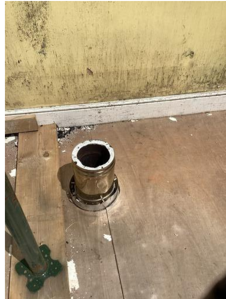
Photograph 68 - Flat 6 (Bed 3) Wood Burning Flue
