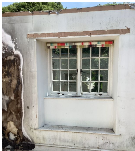
Fig. 11. Photo 3 - Existing timber framed single glazed windows
